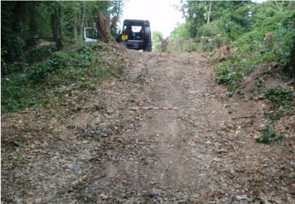
Plate 7. Looking upslope on made-up ground (looking west)
